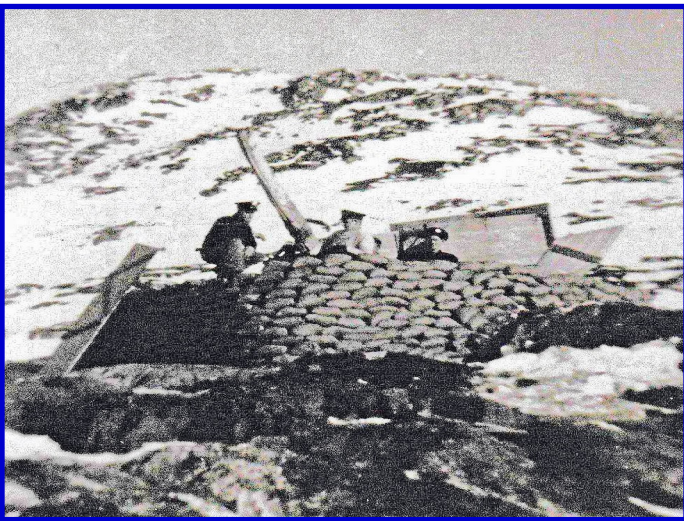
3"/50 gun installed overlooking cryolite mine at Ivigtut. The gun was from CGC NORTHLAND
